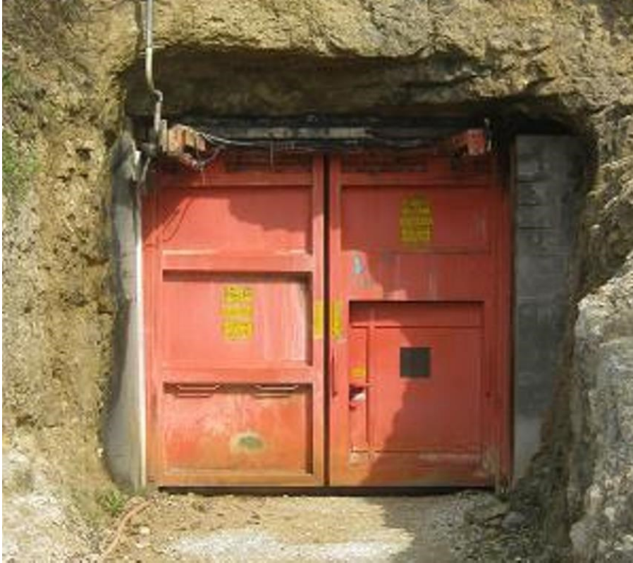
Figure 3.17 Kennedy machine doors
